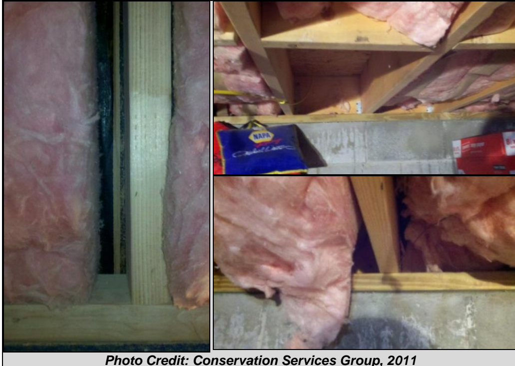
Figure I- 8: Examples of Grade III Insulation Installation
