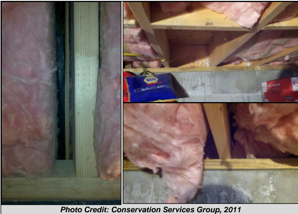
Figure I- 8 shows examples of Grade III insulation in photos taken from this study sample.
