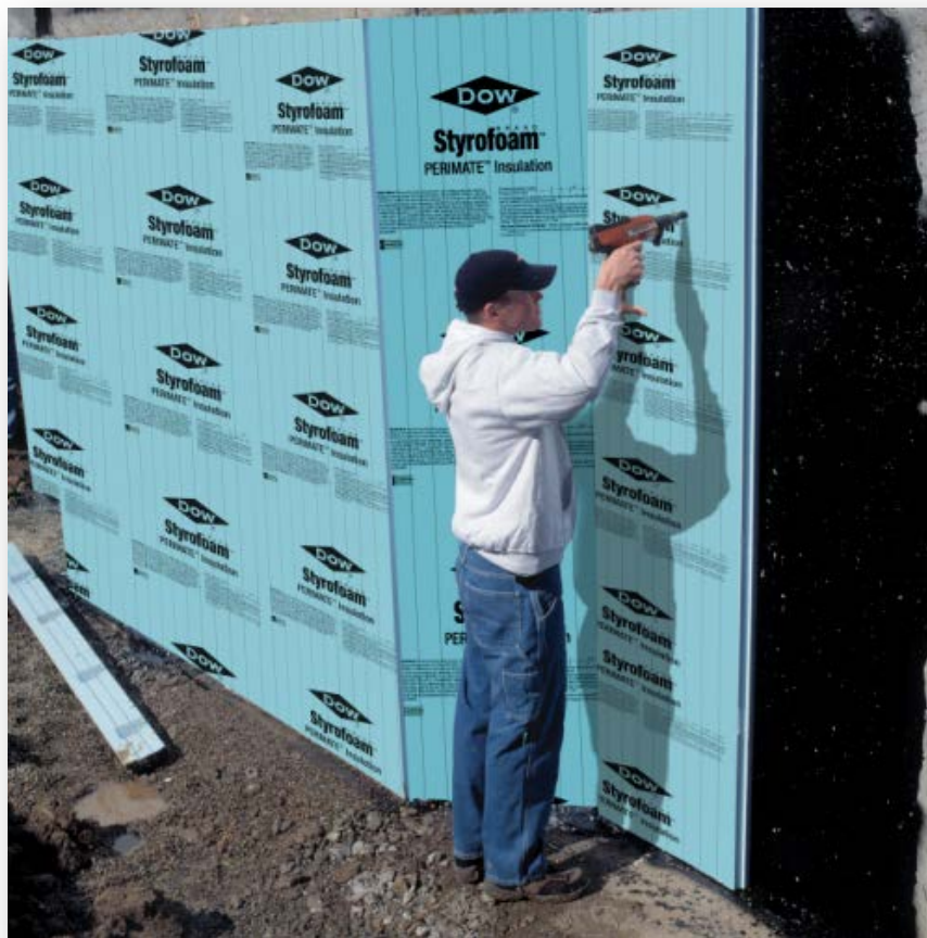
Photo courtesy of Dow Building Solutions
