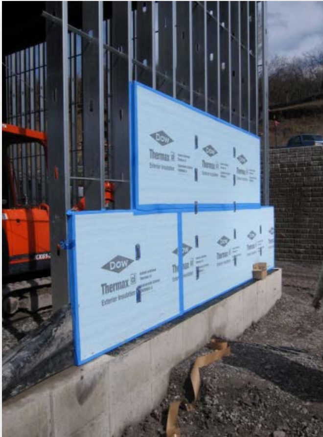
Photo courtesy of Dow Building Solutions
