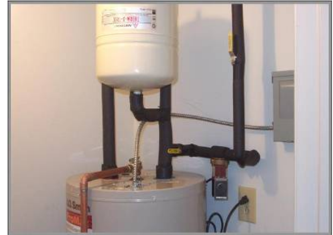
Image courtesy of Ken Baker, K energy
