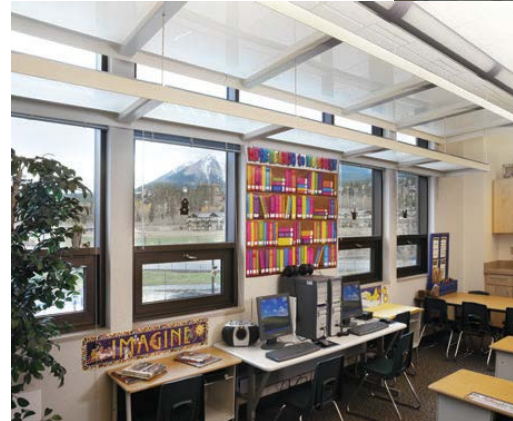
More Efficient Lighting System
