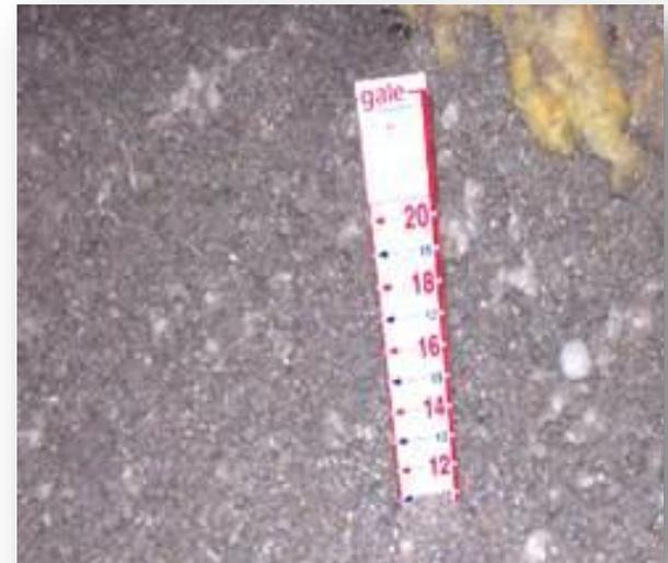
Insulation markers must be installed every 300 square feet and be marked with the minimum installed thickness and affixed to the trusses or joists.
