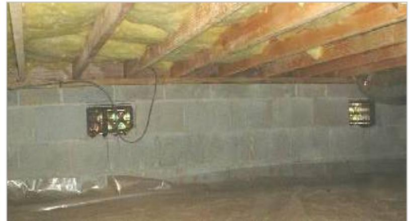
Insulation must maintain permanent contact with underside of subfloor
