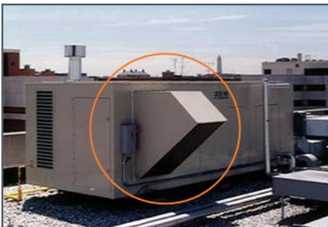
Figure 18: Economizer on a rooftop unit
