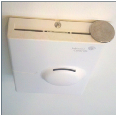
Figure 14: Top view of CO 2 sensor (coin for scale)
