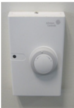
Figure 6: Programmable thermostat, as may be installed in building using packaged HVAC equipment
