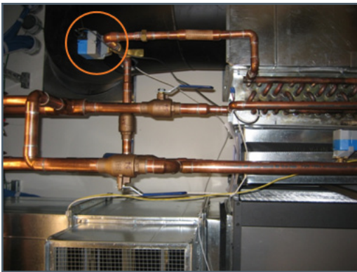
Figure 33: Two position (open/close) valve with electric actuator
