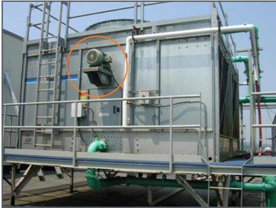
Figure 36: Cooling tower motor — check for connection to VSD
