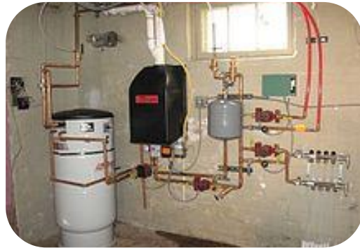
Hot Water Distribution Layout
