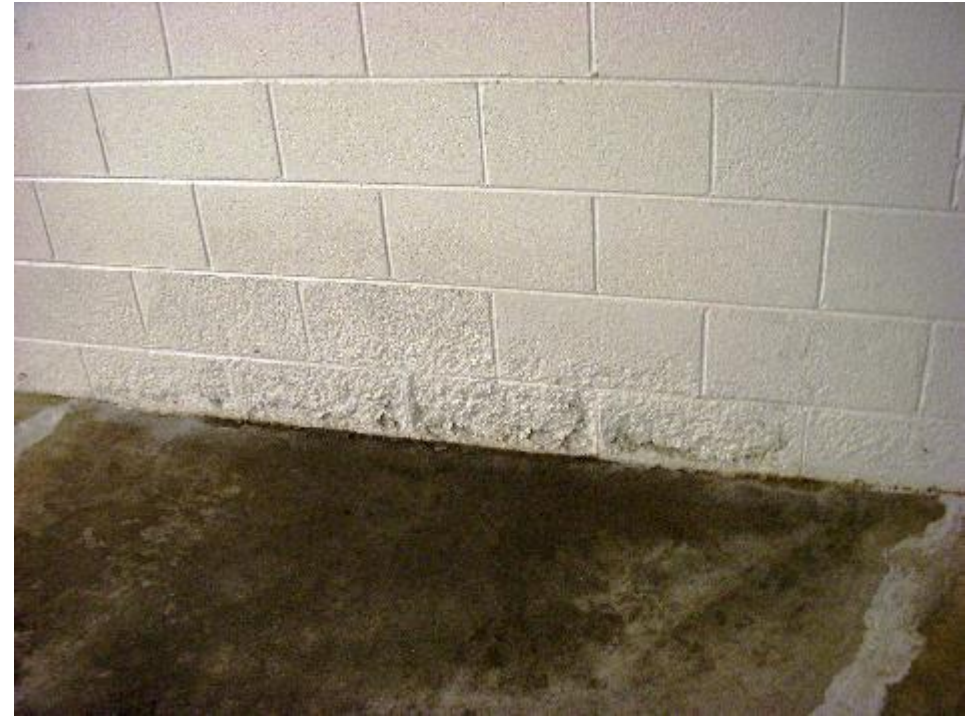
Black mold on concrete floor
