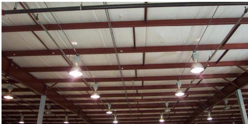
Figure 5012.4 Roof Insulation in Metal Buildings 2
