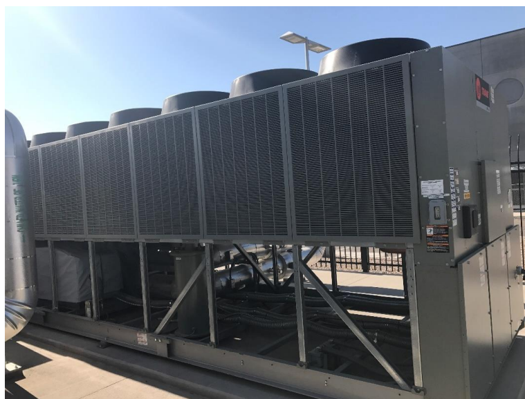
Figure 6007.3 Typical Air-Cooled Chiller
