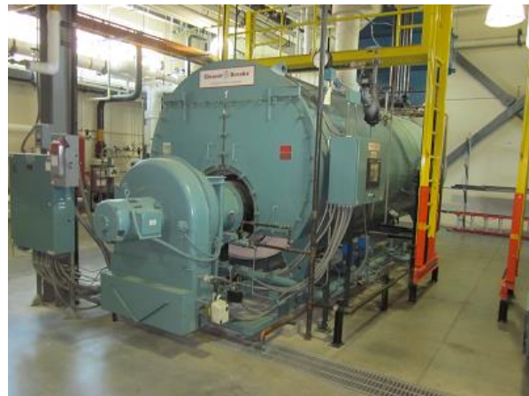
Figure 6005.6 Typical Steam Boiler
