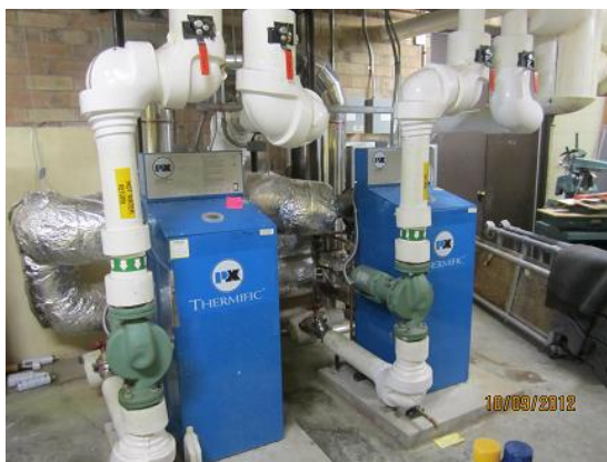
Figure 6005.5 Typical Condensing Boiler
