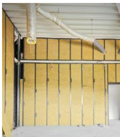
Figure 5018.2 Example of Cavity Insulation 1 Figure 5018.3 Example of Continuous Insulation 2
