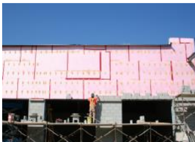
Figure 5018.2 Example of Cavity Insulation 1 Figure 5018.3 Example of Continuous Insulation 2
