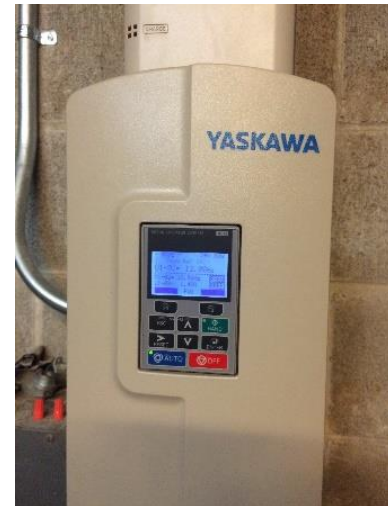
Figure 6109PAS.3 Garage Fan VFD
