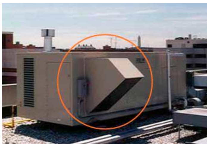
Figure 6066P.1 Outside Air Ductwork for Air Economizer 1
