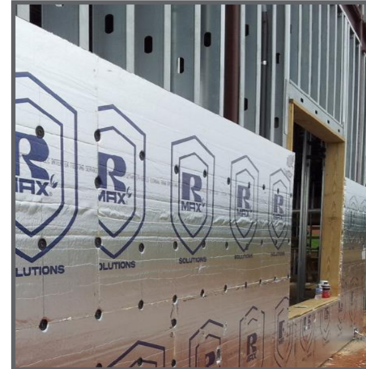
Continuous R-value – used for insulation that is continuous across the structure (e.g., rigid insulation)
