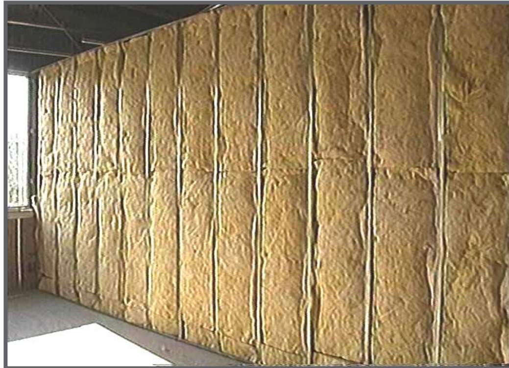
Cavity R-value – used for insulation placed between structural members
