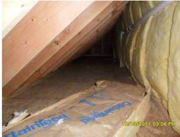
Figure C-3: Grade III Fiberglass Batts—Attic Kneewalls
