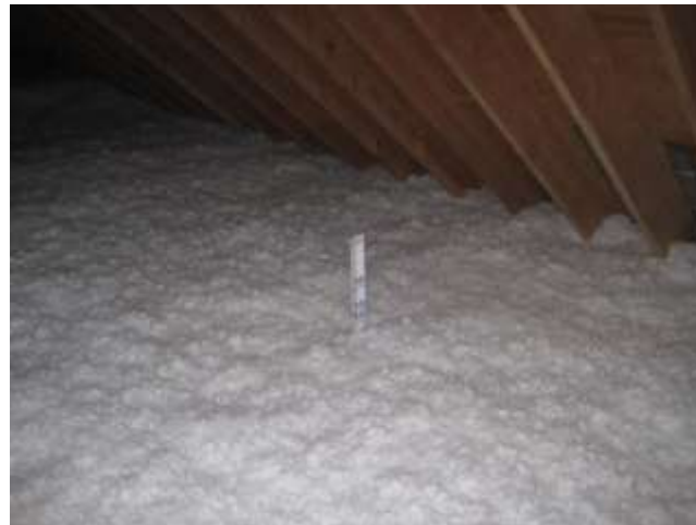
Figure C-6: Grade I Blown Fiberglass—Attic
