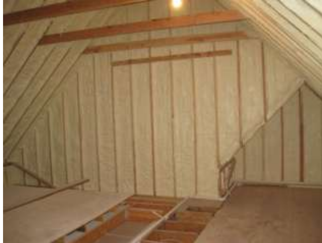
Figure C-1: Grade I Closed Cell Spray Foam—Exterior Walls
