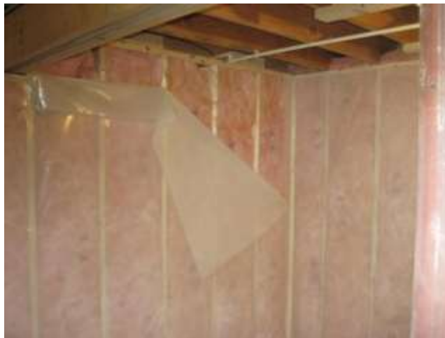
Figure C-2: Grade II Fiberglass Batts—Basement Walls
