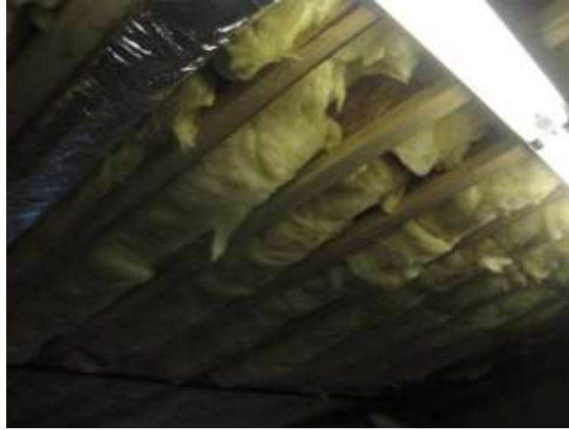
Figure C-5: Grade III Fiberglass Batt—Frame Floor
