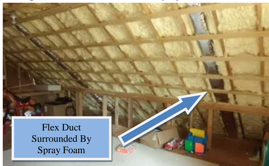
Figure D-14: Roof Rafters with Spray Foam Insulation
