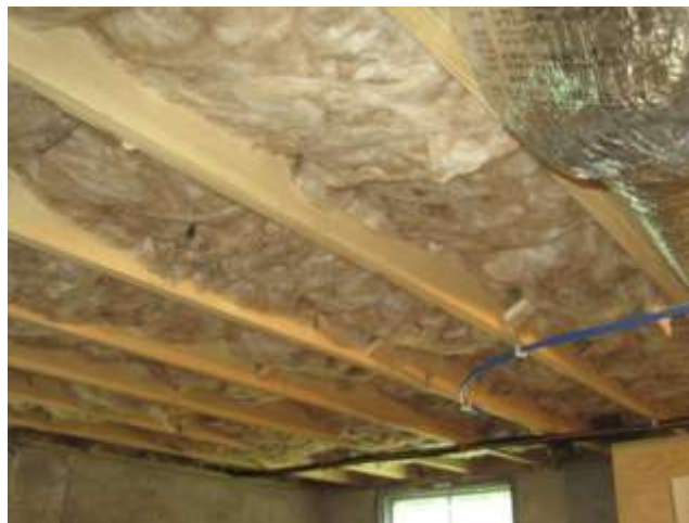
Figure C-4: Grade II Fiberglass Batts—Frame Floor
