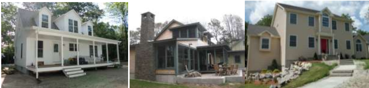
Figure 1-3: Examples of Inspected Homes
