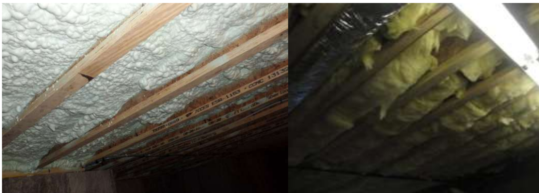
Figure 1-4: Example of Grade I and Grade III Floor Insulation Installation
