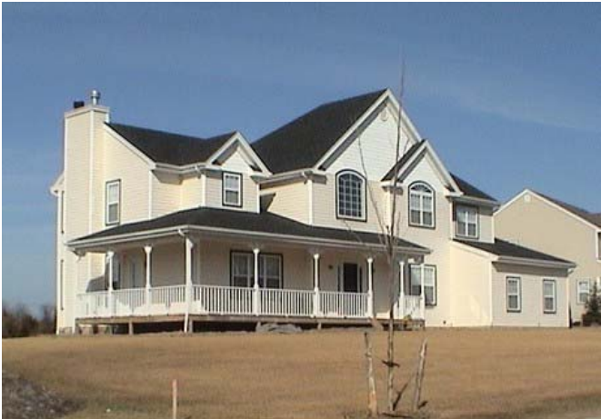
Figure 3 Representative Long Island Single-Family Detached Home
